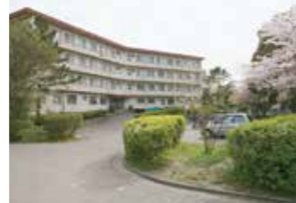
五十嵐寮 A棟・B棟 Ikarashi Hall Buildings A and B
